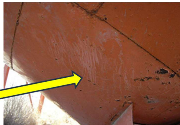
Teeth marks of sheep on the side of the field bin. Lead levels on paint very high.
