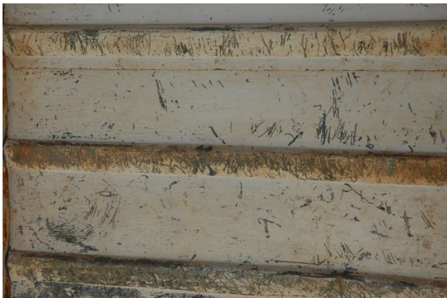
Sheep chewing paint off shed which has high levels of lead (74,202 ppm).
